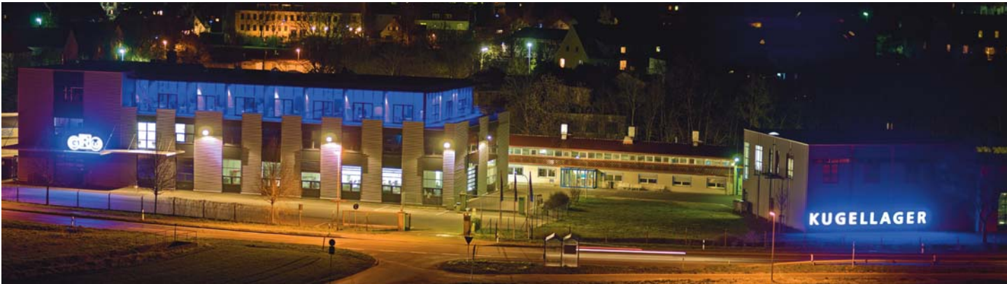
Headquarter and production site at Rimpar
